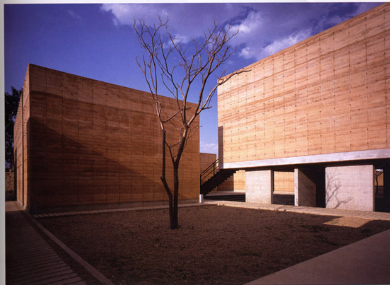
Oaxaca School of Arts, Tallerdearquitectura- Mauricio Rocha, Gabriela Carrillo, Carlos Facio, Rafael Carrillo, 2007-2008, Oaxaca, Mexico. Courtesy of Louise Noelle
